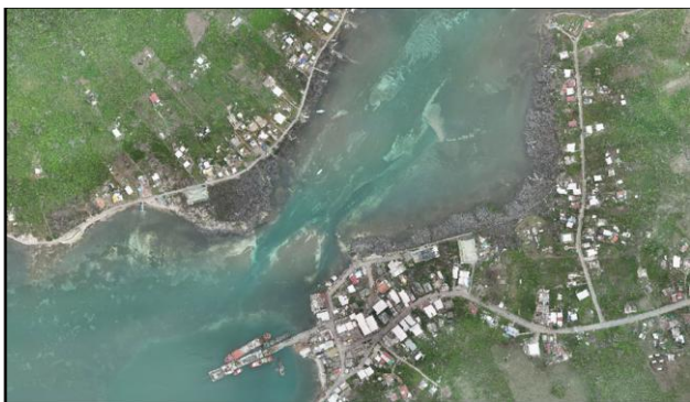
Figure 4. Road infrastructure loss
